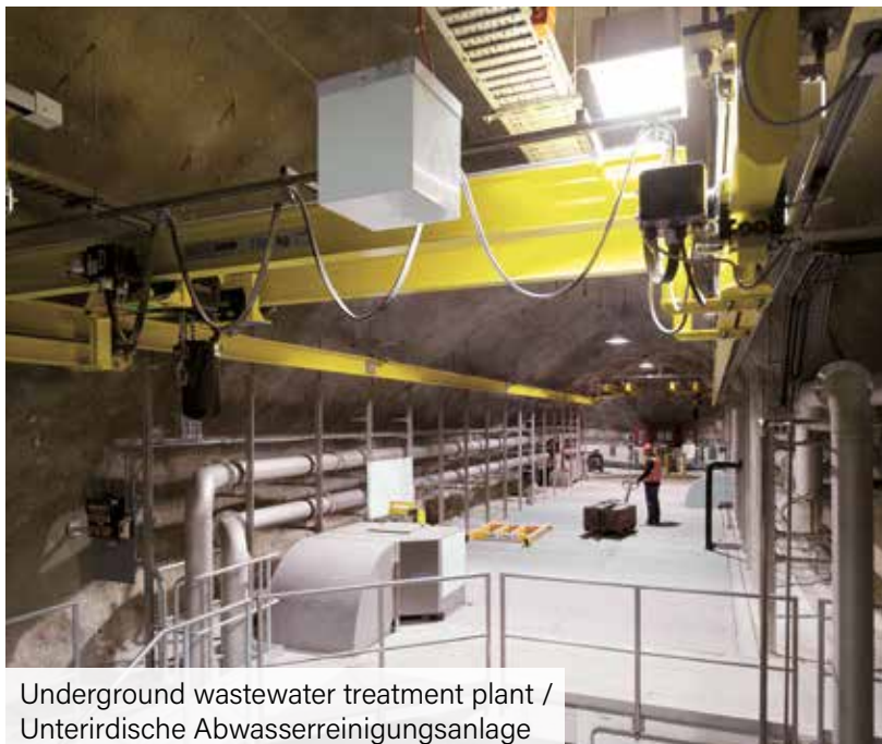
Control cabinet installation by Rittmeyer / Schaltschrankinstallation von Rittmeyer
